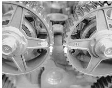
Fig. 23: Rotate the crankshaft until the timing marks (arrows) on the camshaft sprockets align with each other
